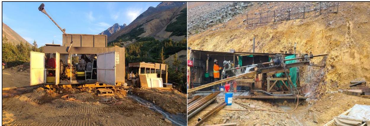
Figure 10-2: Typical drill set up at Berg
