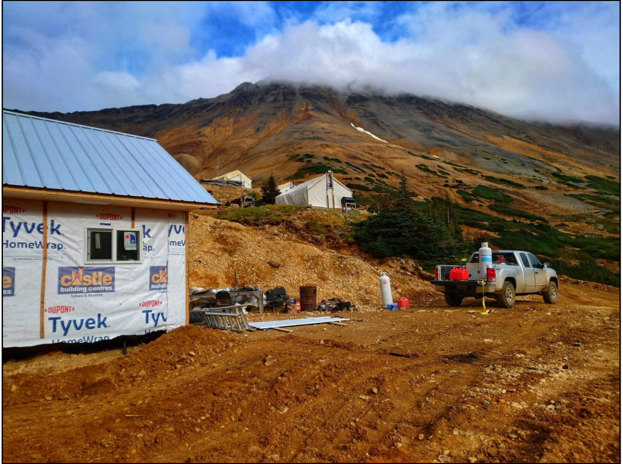
Figure 3. Berg camp construction progress.
